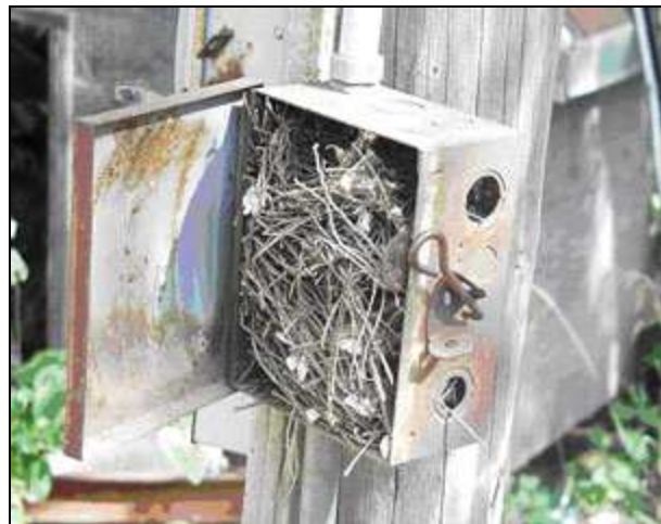
Picture #2: Pull box between house and corn bins with nesting materials.
