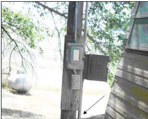
Picture #1: Pull box with conduit running to grain bins.
